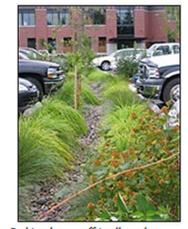
Parking lot runoff is allowed to infiltrate through a vegetated bioretention area
